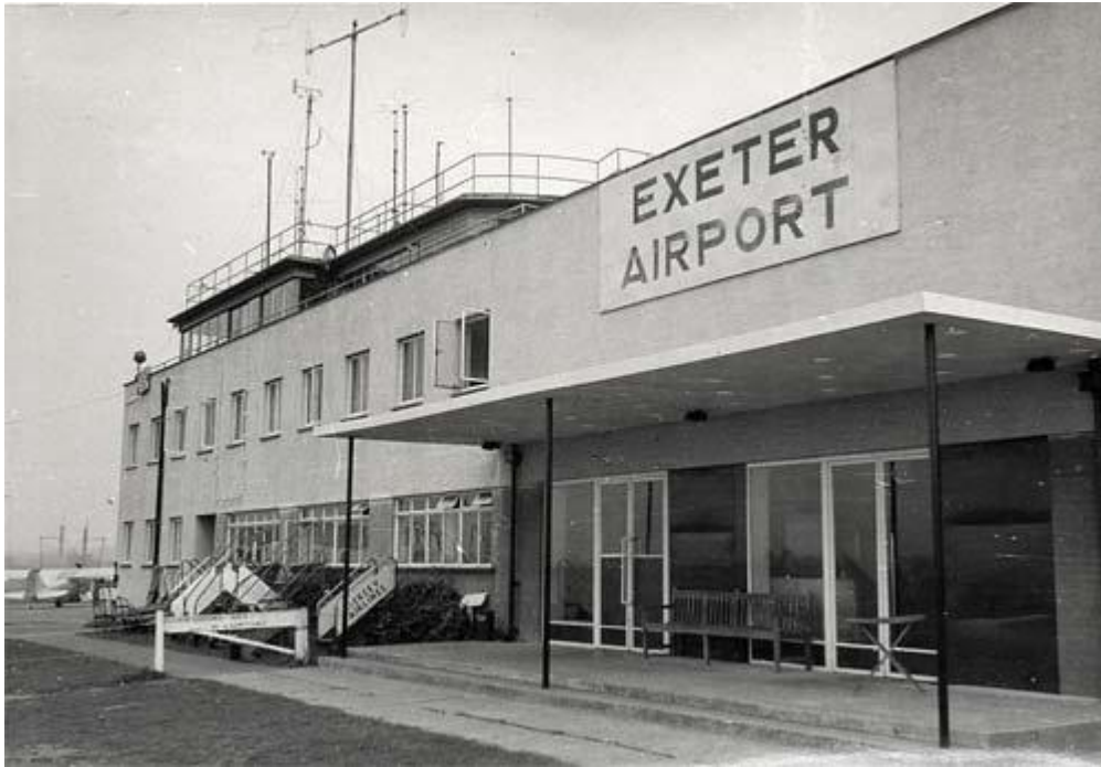
Original terminal building
